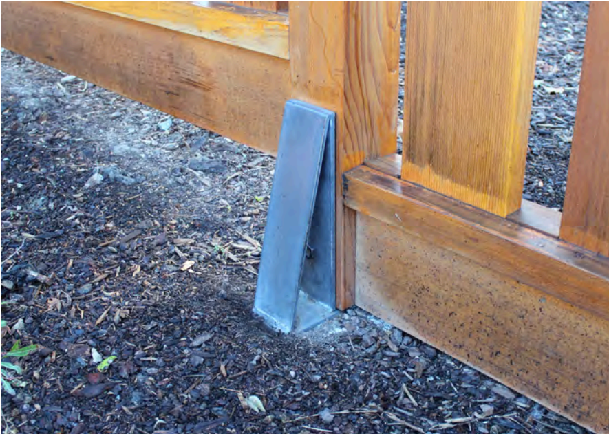
Interior view close-up
