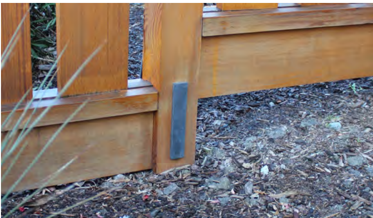
Street view close-up
